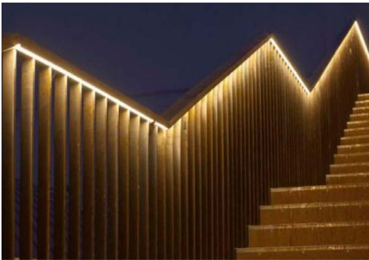
Low level diffused lighting on new stair connection handrails to help guidance and wayfinding
