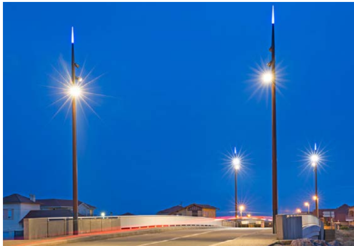
Improved lighting locations across bridge. Highlevel lighting upgraded to LED.
